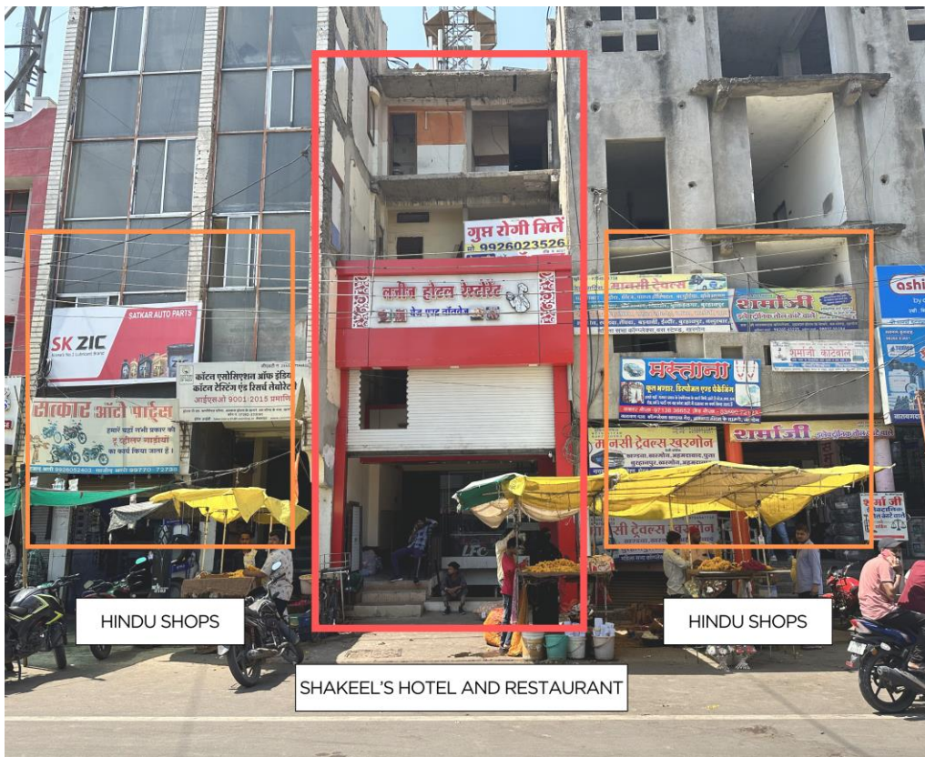
Khargone, Madhya Pradesh: Shakeel's hotel and restaurant was the only shop to be demolished while the neighbouring Hindu shops were left untouched.
